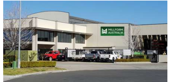
MILLFORM SYDNEY OFFICE & MANUFACTURING FACILITY
