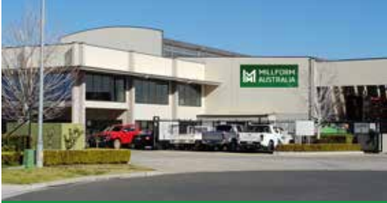
MILLFORM SYDNEY OFFICE & MANUFACTURING FACILITY
