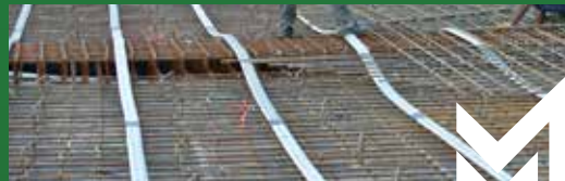
SLAB & SPIRAL DUCT
