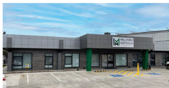
MILLFORM ALBURY OFFICE & MANUFACTURING FACILITY
