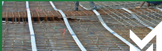
SLAB & SPIRAL DUCT
