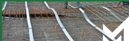
SLAB & SPIRAL DUCT
