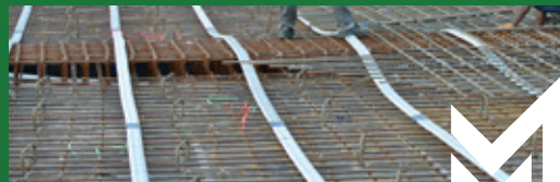
SLAB & SPIRAL DUCT
