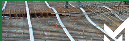
SLAB & SPIRAL DUCT
