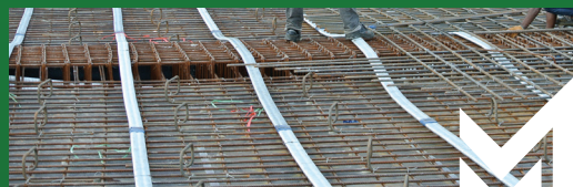
SLAB & SPIRAL DUCT
