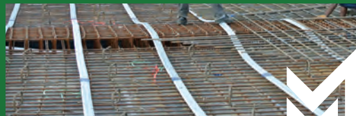
SLAB & SPIRAL DUCT
