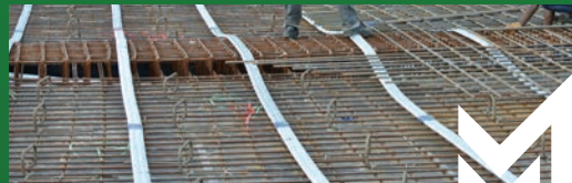
SLAB & SPIRAL DUCT
