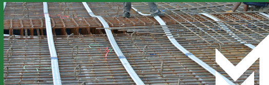
SLAB & SPIRAL DUCT
