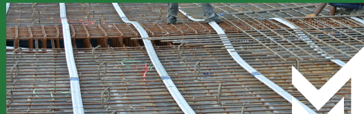
SLAB & SPIRAL DUCT
