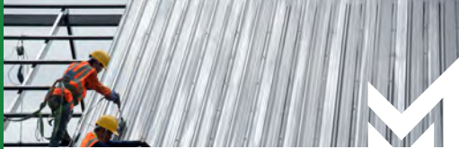
CORRUGATED SHEET METAL
