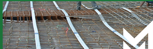
SLAB & SPIRAL DUCT
