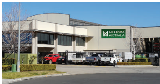
MILLFORM SYDNEY OFFICE & MANUFACTURING FACILITY
