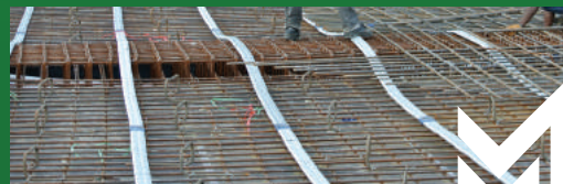
SLAB & SPIRAL DUCT
