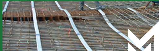
SLAB & SPIRAL DUCT
